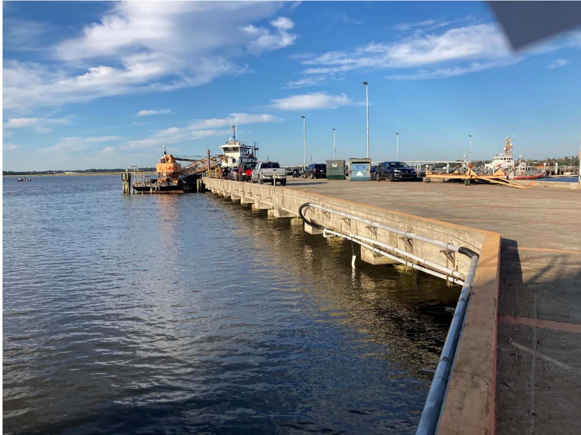
2. Coast Guard Pier looking at southwest toward the Ashley River
