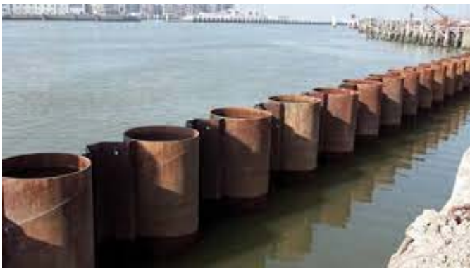
View of Constructed Combo Wall Substructure
