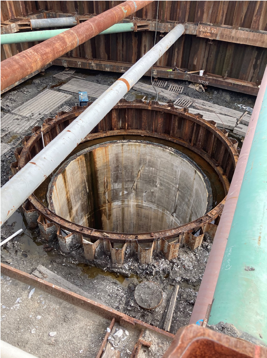
150' deep wet well shaft in shored excavation
