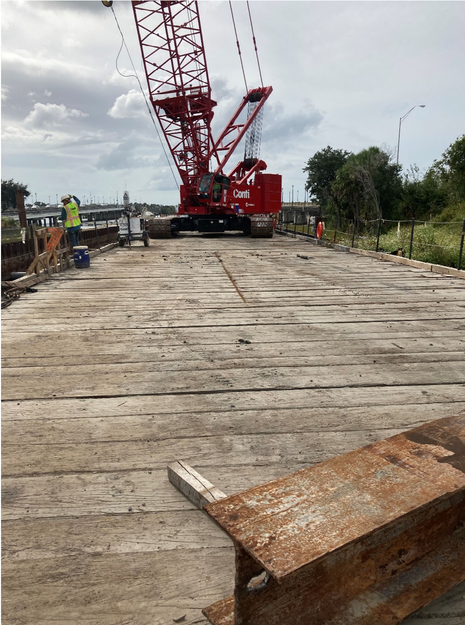
View of trestle deck and crane
