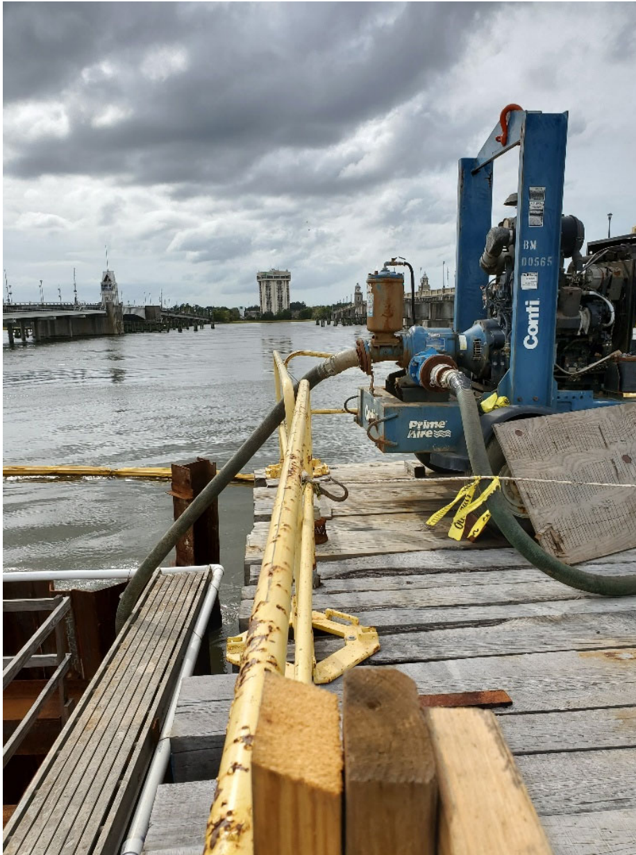
Dewatering pump – we would not need this for floodwall construction
