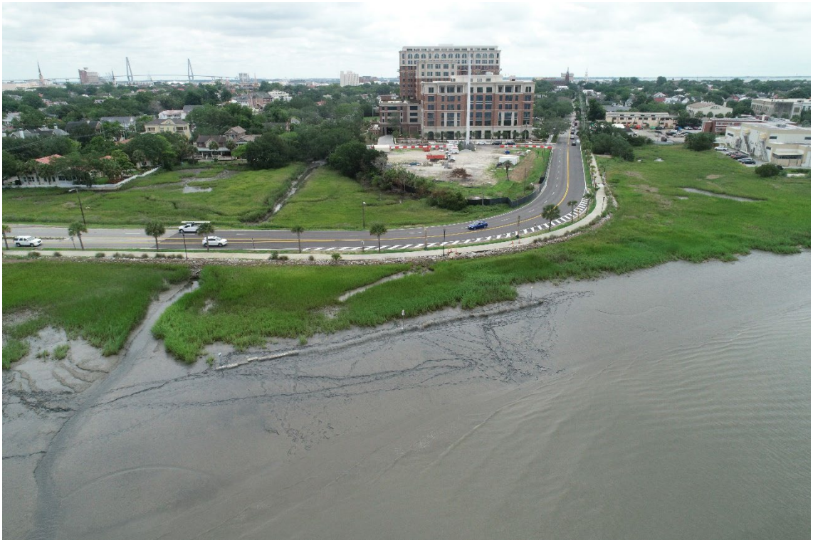
Figure 6.3. Recently completed segment of living shoreline constructed by SCDNR from manufactured wire reef sills along the Ashley River near the corner of Lockwood Blvd. and Broad Street. Note the location from the low tide waterline and proximity to the vegetated shoreline. Source: photo courtesy of SCDNR.
