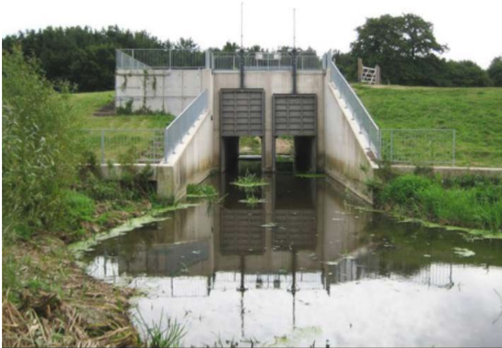
Figure 5.6.11: An Example of a Pair of Sluice Gates (Photo courtesy of USACE Norfolk District)
