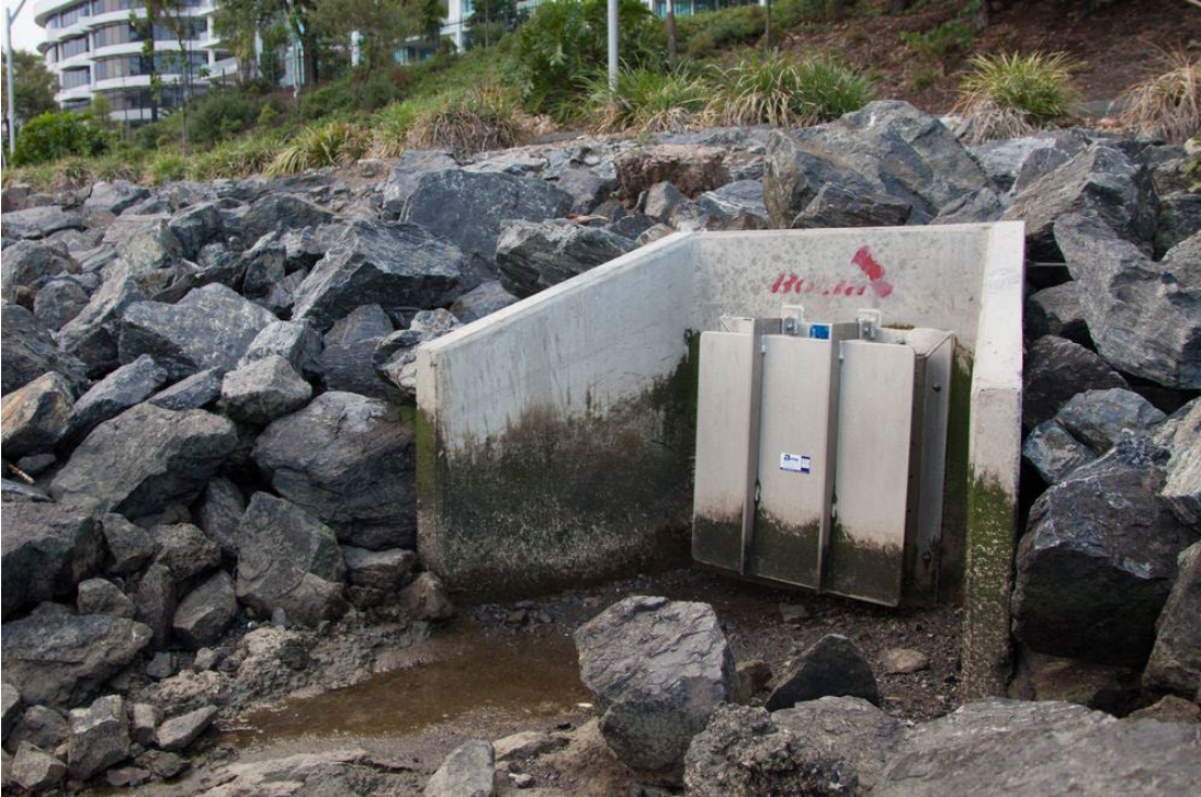
Figure 5.6.6 Example of Flap Gate Style Check Valve (Photo courtesy of USACE Norfolk District)
