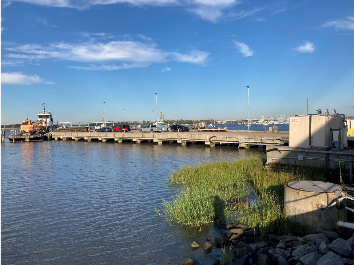
3. Coast Guard Pier looking at downstream side
