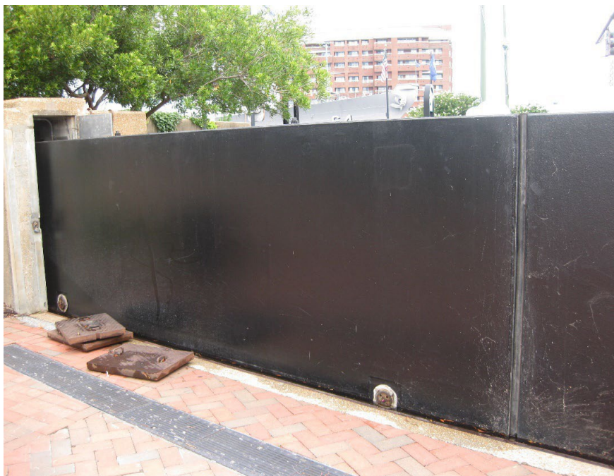
Figure 5.6.4: Slide Gate Example (Photo courtesy of USACE Norfolk District)
