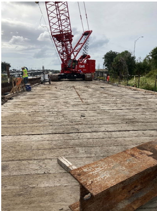
VIEW FROM DECK OF WORK TRESTLE
