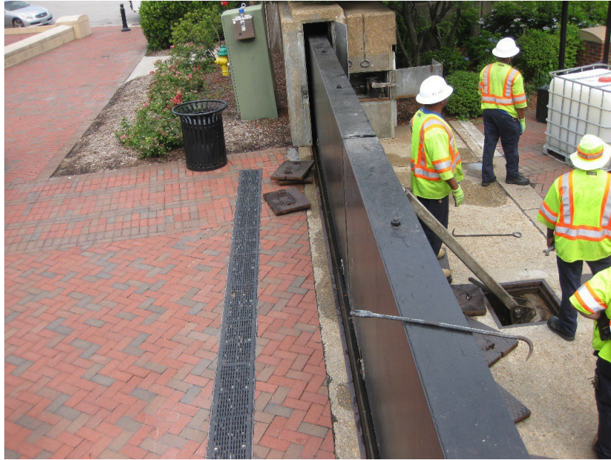
Figure 5.6.3: Slide Gate Example (Photo courtesy of USACE Norfolk District)
